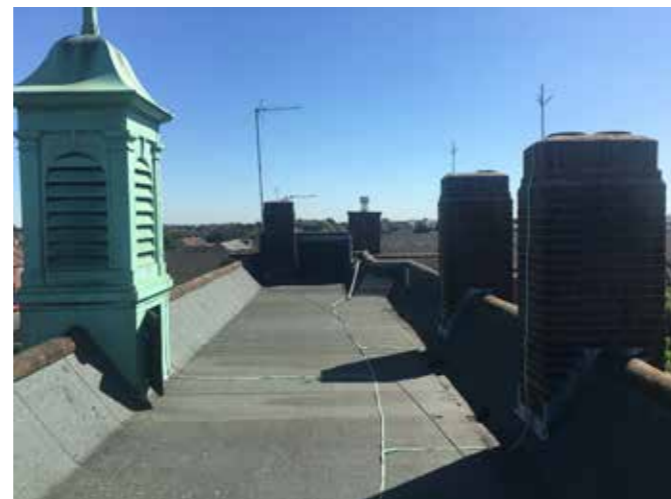
View from the roof showing cupola and chimneys
