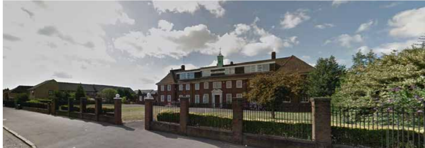
View from Goresbrook road looking South East
