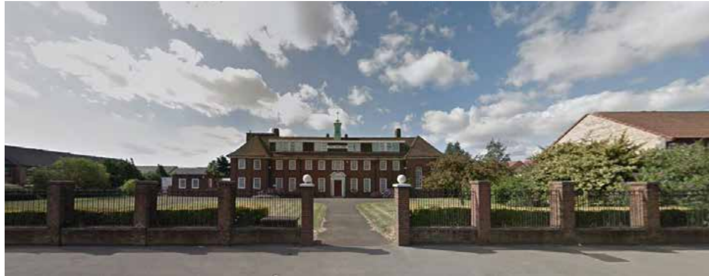
View from Goresbrook road looking South
