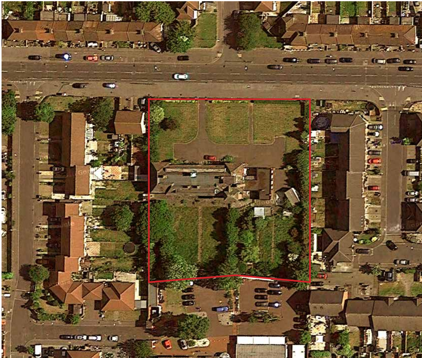
Aerial view of site with red line indicating site boundary.
